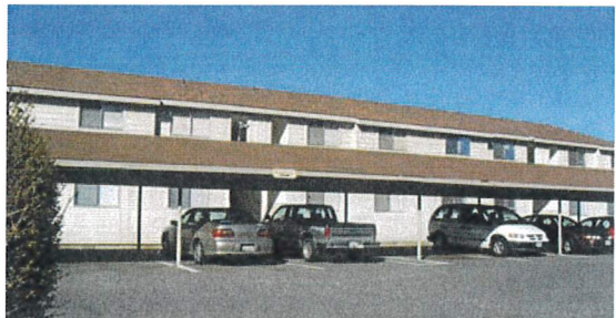
Long, continuous carport in the front.
