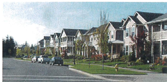
Consistency in the roofline and building form.
