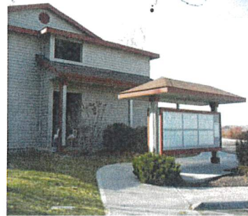
Mailbox consistent with the main structure.
