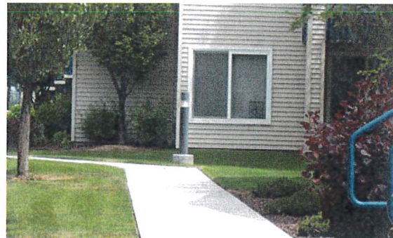
Bollard lighting on walkways.
