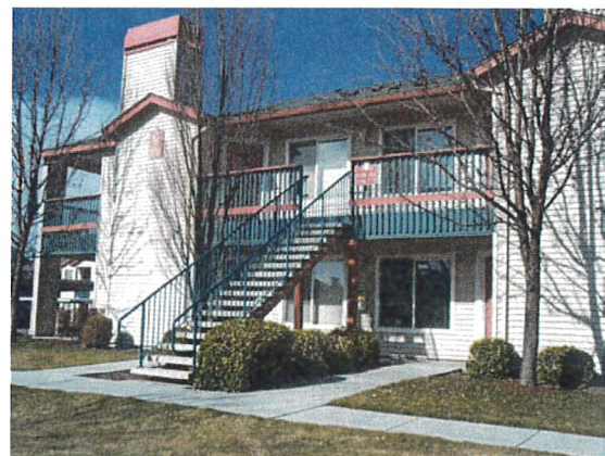
Open, visible entry stair and corridor.
