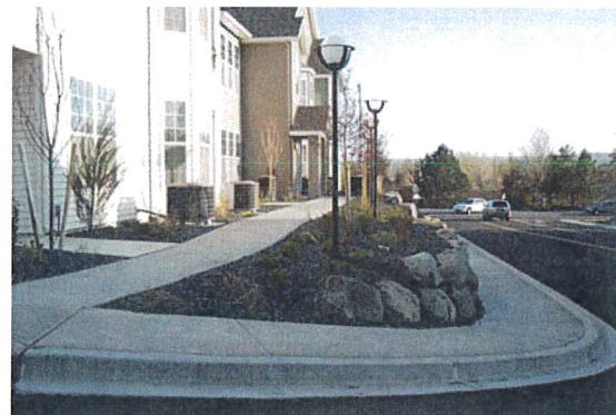
Safe pedestrian access along with vehicular access.
