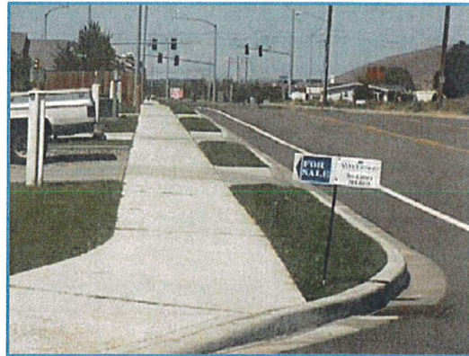
No street trees and narrow planting strip.
