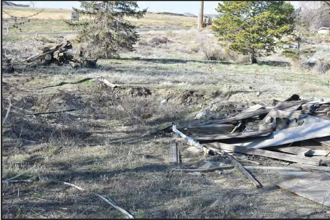
Figure 6. Overview of demolished shed 1, view to the west.
