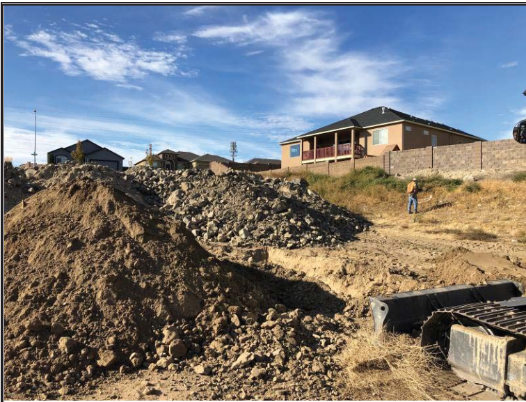
Recently placed stockpiles of rocky soil material in southern portion
