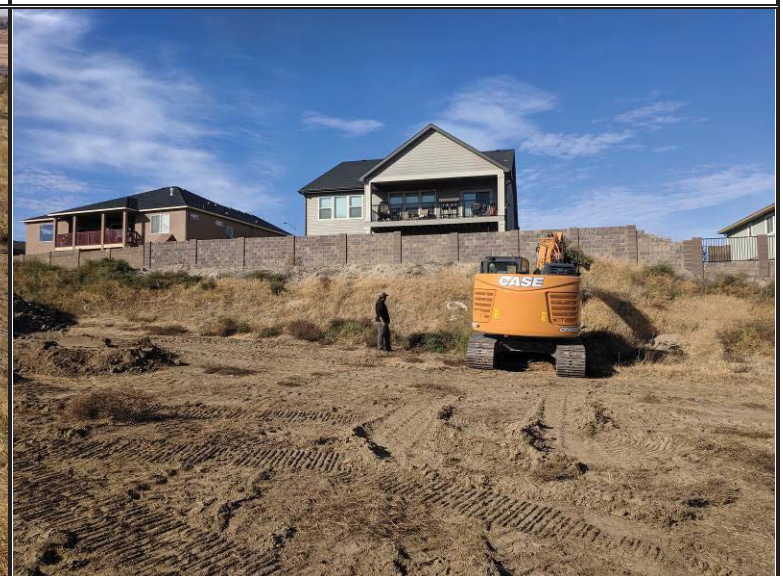
Excavating test-pit TP-2 in southwestern portion of site, looking west
