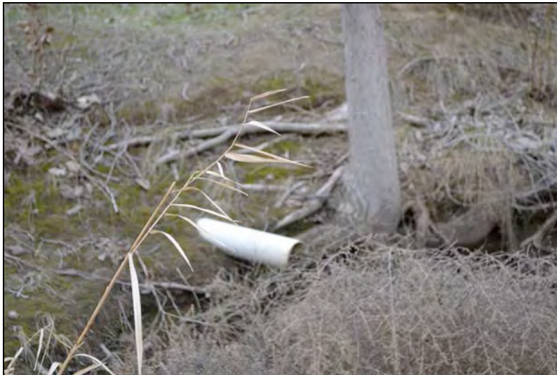
Photo B14: This photo is showing one of the two pipes that allow water flow into the pond; both are located in the southeast corner area of the pond.
