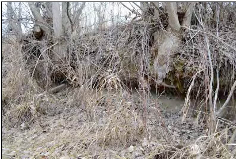
Photo B8: There is evidence of extensive erosion through Area B; the roots of cottonwood trees along the banks of the ravine are exposed through most of the area.
