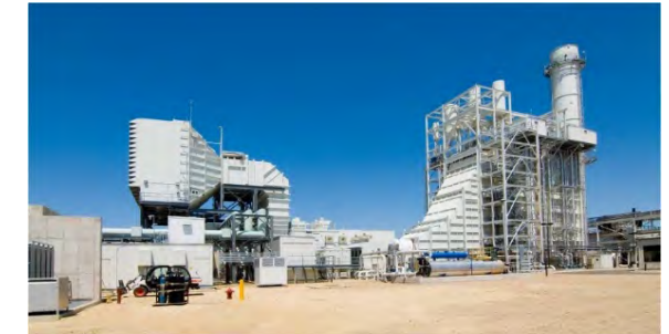
Natural Gas CCCT Plant
