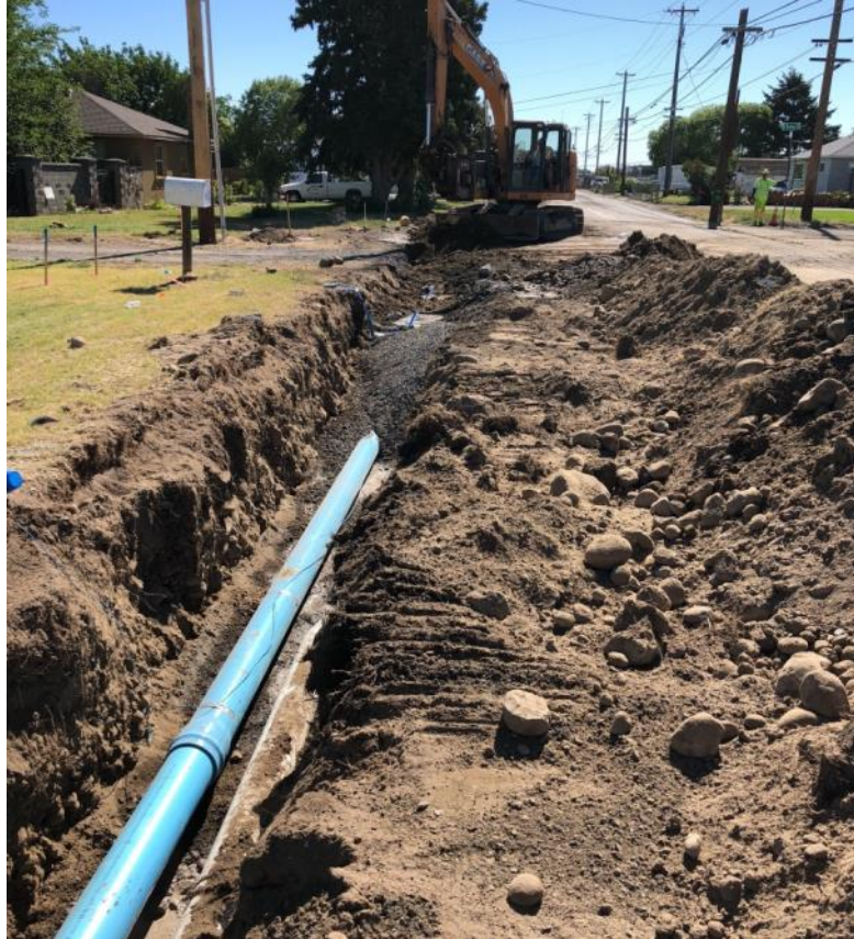
Waterline Installation
