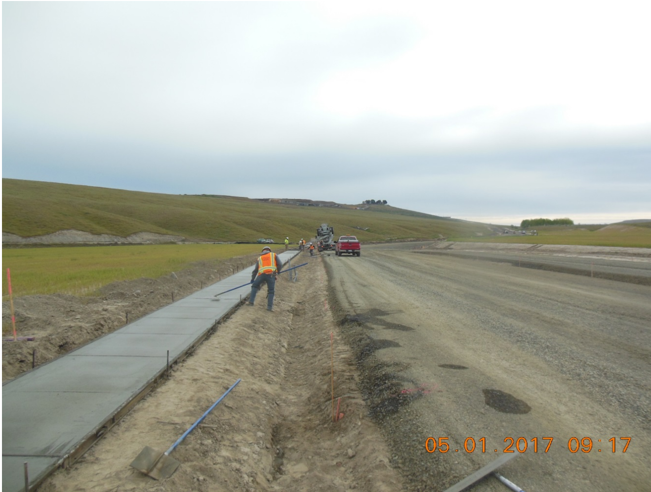
Sidewalk being poured adjacent to the Southcliffe Commercial area.
