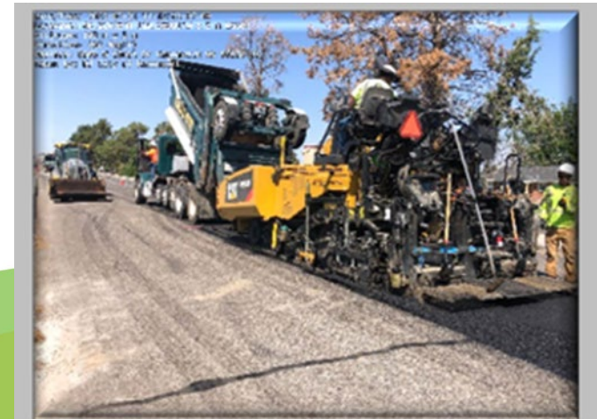
Overlaying W. 10 th Ave.
