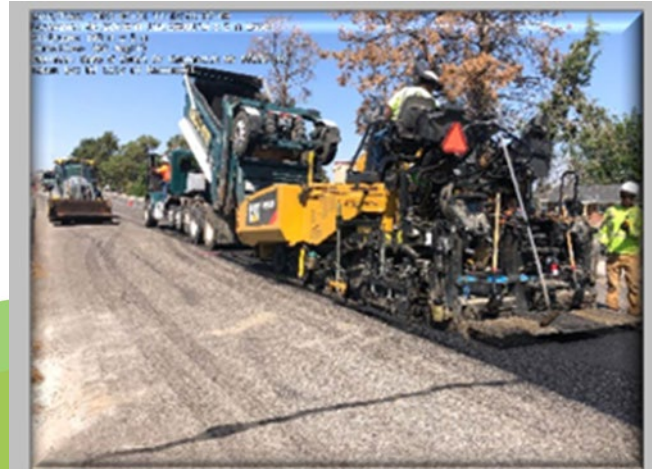
Overlaying W. 10 th Ave.
