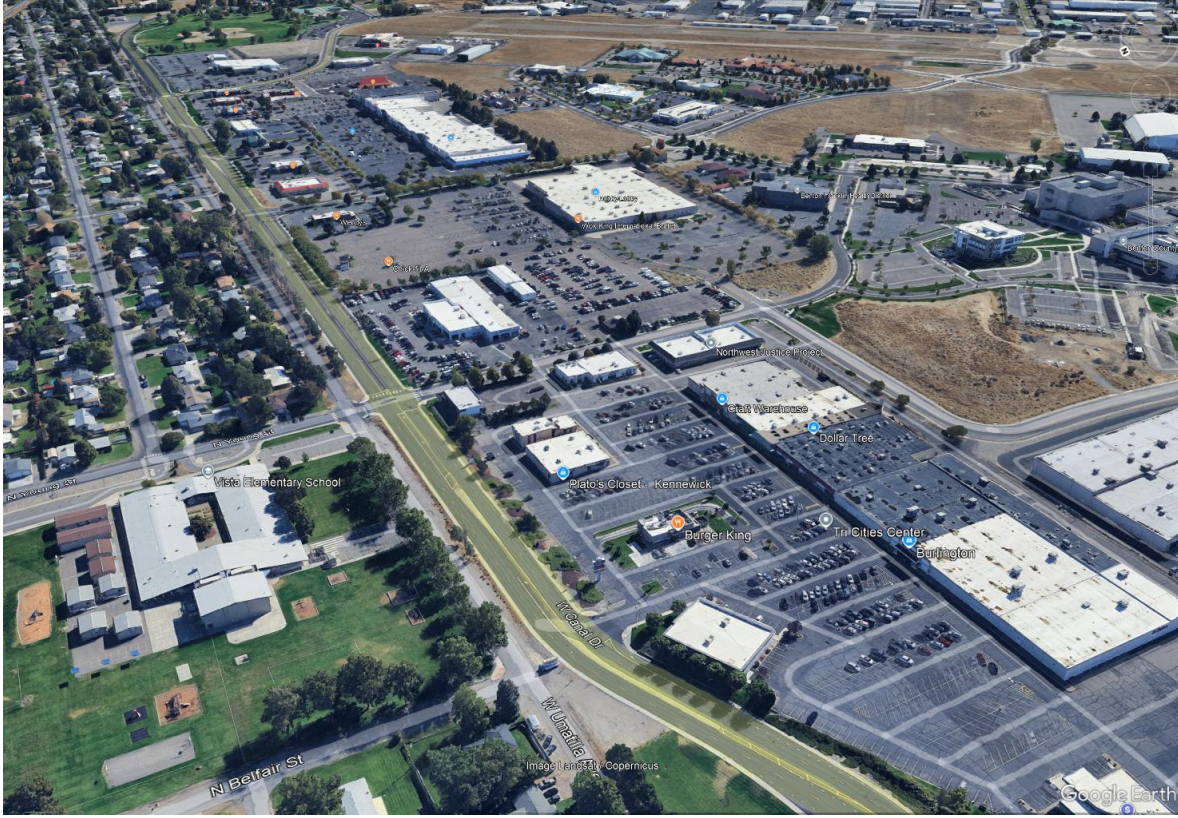
W. Canal Drive, looking east
