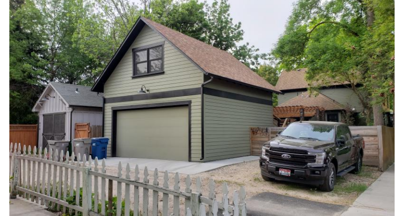
ADU above a garage in Boise, ID
