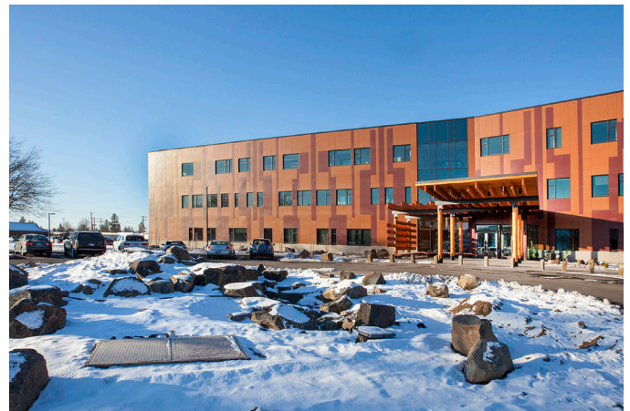
In addition to Richland City Hall, Architects West and Opsis partnered on The Confederated Tribes of the Colville Reservation, Lucy F. Covington Tribal Government Center, which brought 52 agencies into a single 160,000 sf building.
