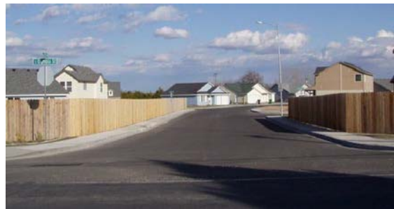
Fence on the edge of the sidewalk
