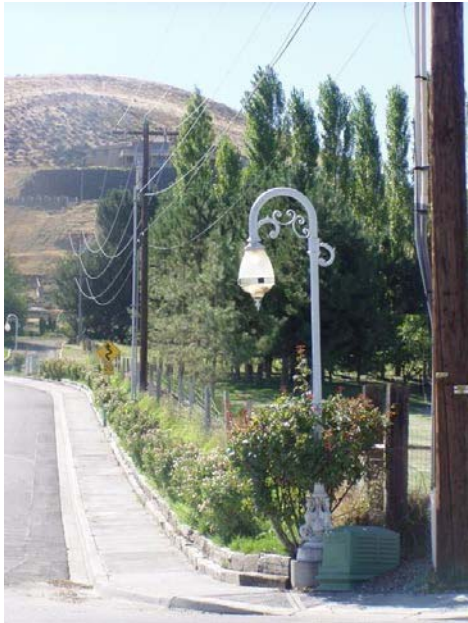
Meadow Hills subdivision street lights
