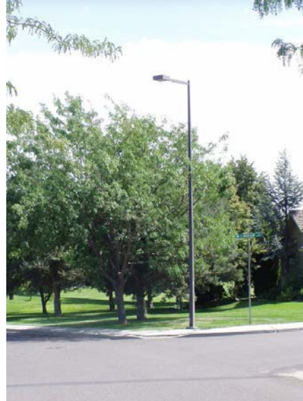
Street light at Canyon Lakes
