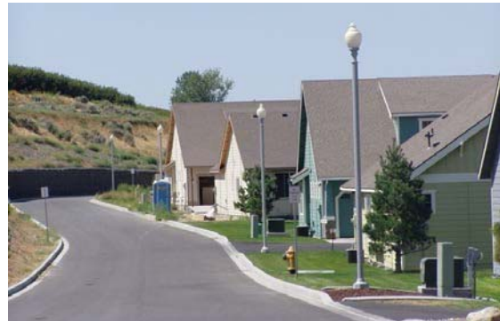
Street light at PineWood neighborhood
