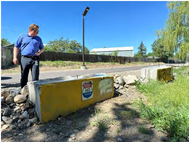
Figure 7. Barricaded local street access to the Highland Feed Canal Pathway at A Street
