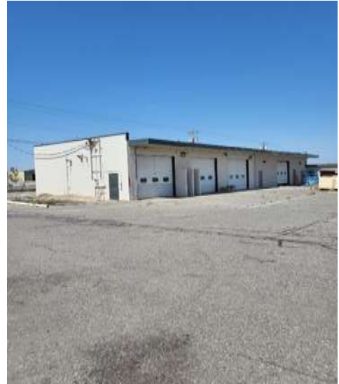
Figure 8-1. Benton County MRW Facility
