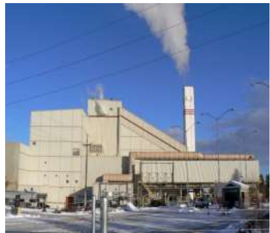
Figure 9-1. City of Spokane Waste-to-Energy Plant
