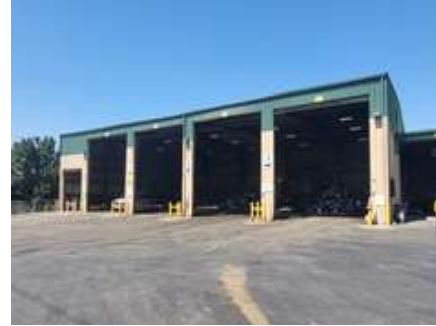
Figure 4-2. WM Kennewick Transfer Station
