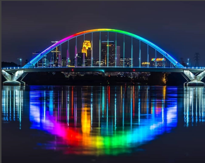
The Lowry Bridge located in Minneapolis, MN
