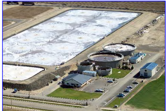
Two, 1.5 MG AWWA D110 Type III prestressed concrete tanks constructed in Sunnyside, WA.
