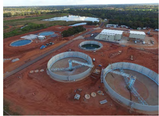
Two ~1.0 MG AWWA D110 Type III prestressed concrete tanks built for the Residuals Handling Facility at the Draper WTP in Oklahoma City.
