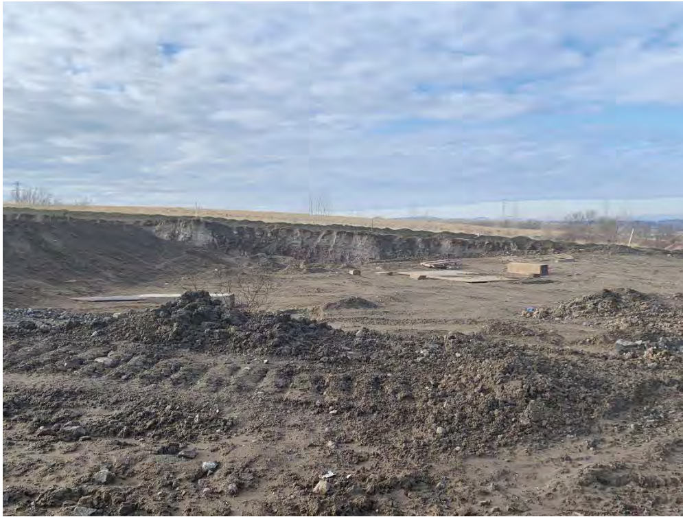
Figure 12. Overview of portion of the project area graded and excavated - note the construction material (Aspect: West).
