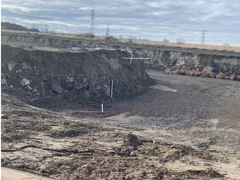
Figure 13. View of portion of project area excavated with white PVC pipes sticking out of the soil profile wall in the left of the frame (Aspect: Southwest).
