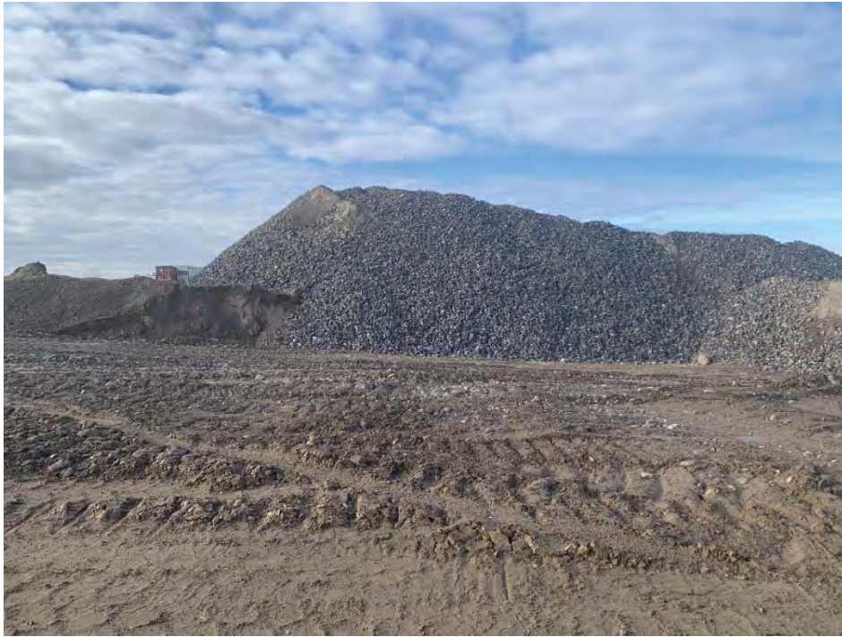
Figure 21. Overview of fill pile in the northern portion of the project area (Aspect: West).
