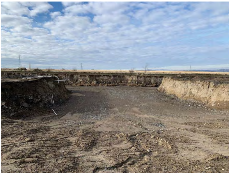
Figure 7. Overview from the southeastern portion of the project area that has been excavated and graded (Aspect: West).
