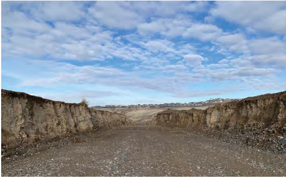
Figure 10. Overview of portion of the project area excavated (Aspect: North).
