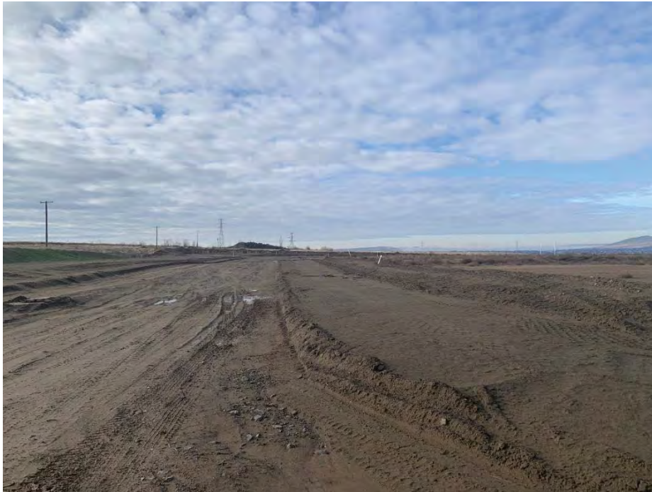
Figure 15. Overview of southern portion of the project area - note the area graded for the placement of a road (Aspect: West).
