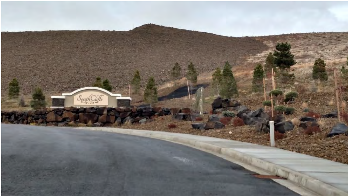
(Southcliffe subdivision on Thompson Hill – Use of riprap for slope stabilization.)
